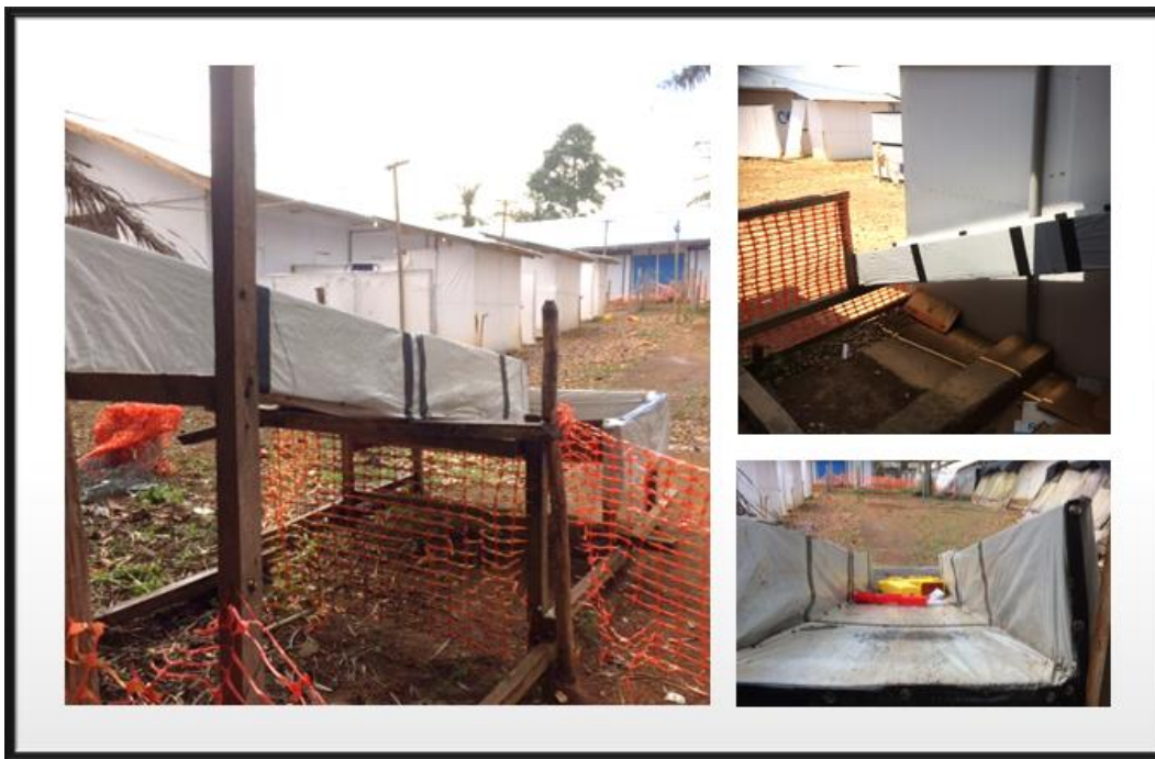
Photo of slides used in an ETU for food provision from low-risk to high-risk zones. (Photo Credit: Mija Ververs)
